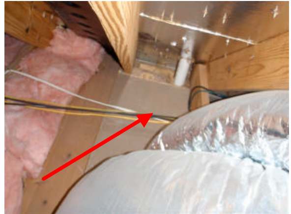
Ensure insulation is maintained a minimum of 3 inches and wood a minimum of 1 inch from around all recessed lights to reduce possible fire hazard.
