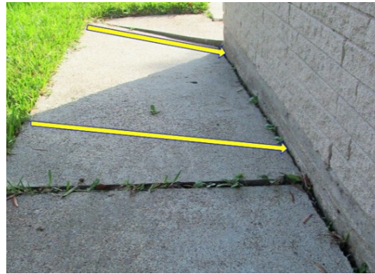
Should slope away from the foundation
