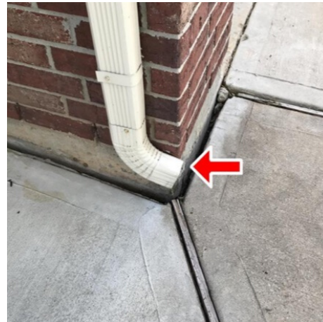
Should slope away from the foundation
